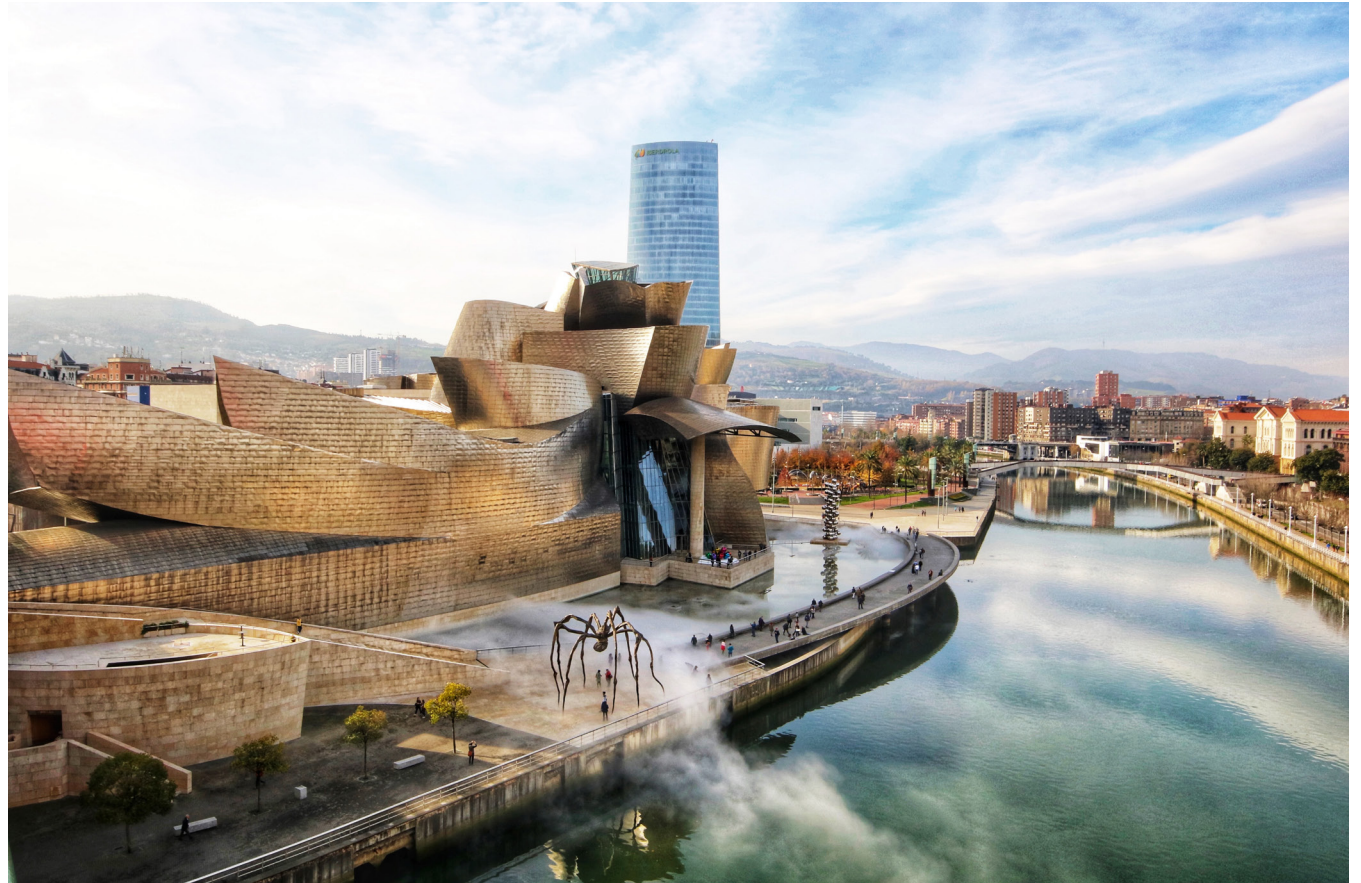
Figure 2.2: Guggenheim Museum. (source: link )
