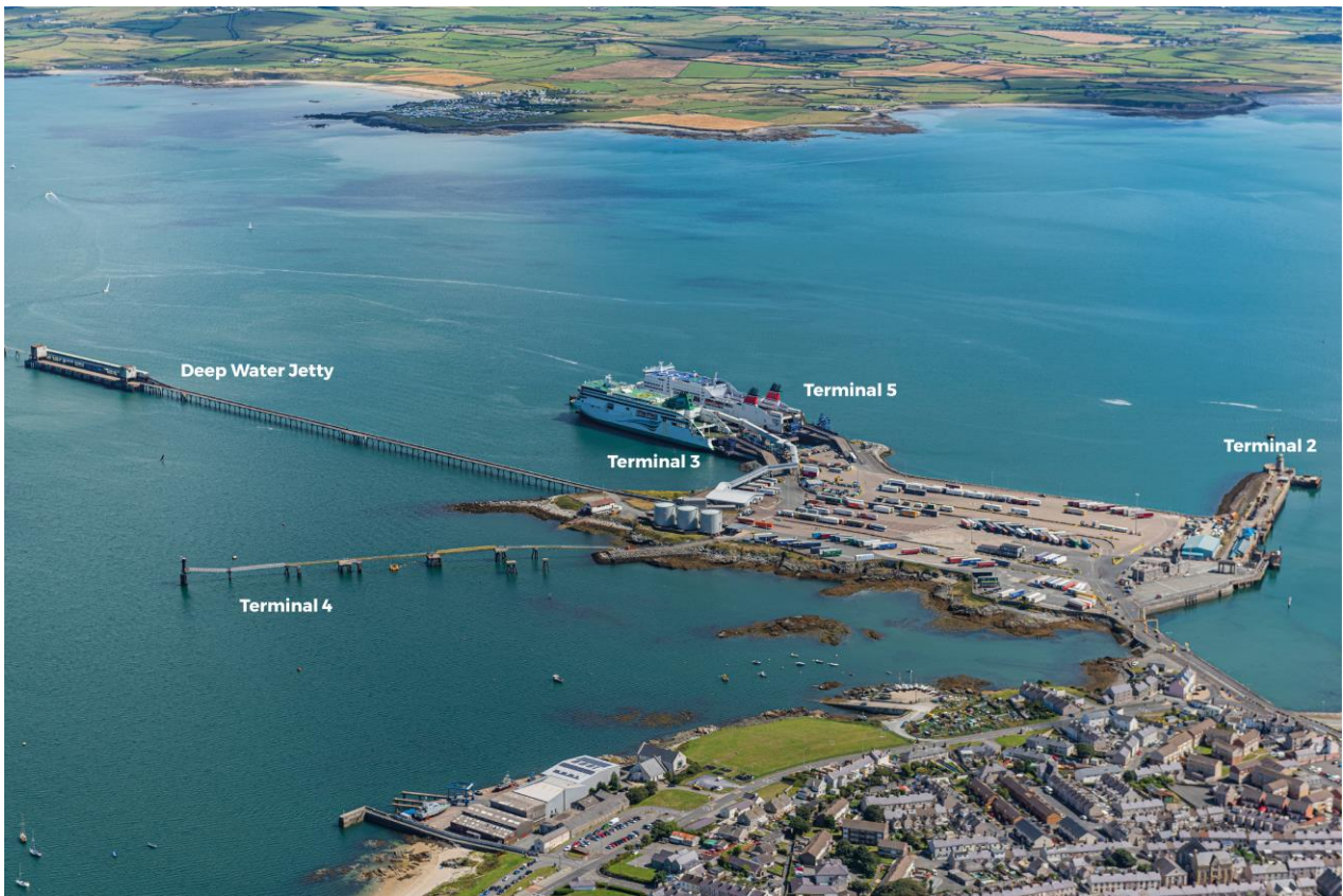
Figure 1 A birds-eye view of a section of Holyhead port
